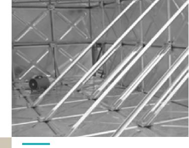
There are 4 different types of metal stays with two different classification , this is best described as tiers 1 to 4 and either diangular or horizontal - Tiers 1 and 2 are manufactured out of 70 x 70 x 6 angles with 8 mm base plates and tiers 3 to 4 are 60 x 60 x 6 with the same 8 mm base plate
